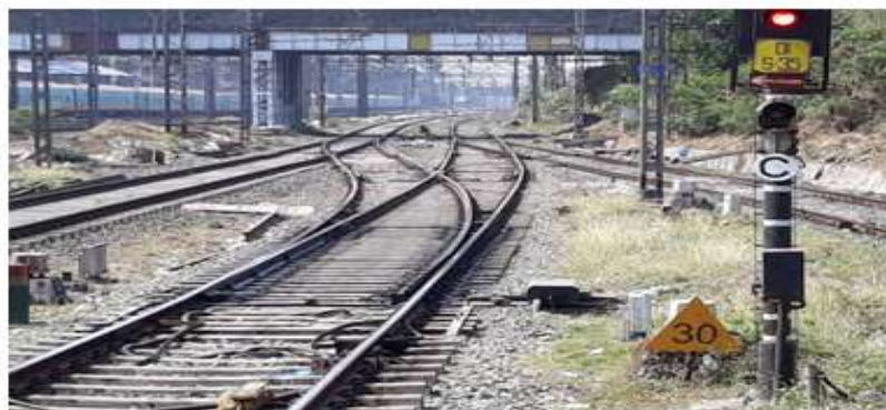
Figure 3: Automatic Track Switching
