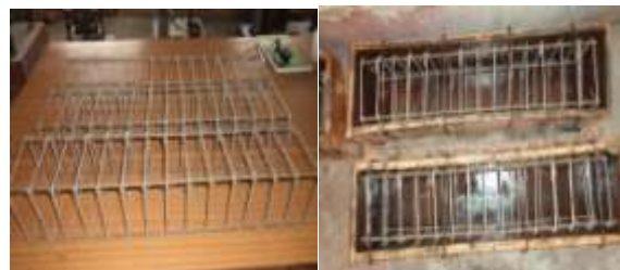
Fig. 2.6 Reinforcement cage filled in moulds
