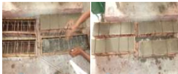
Fig. 2.7 Casting of beam moulds
