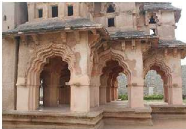
Fig.2 Use of stone Arch in Vijayavittala Temple of Hampi-Vijayanagara
