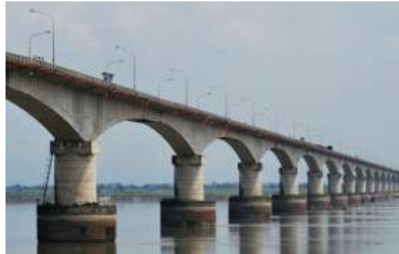
Fig.4 Use of Arch in Bridge
