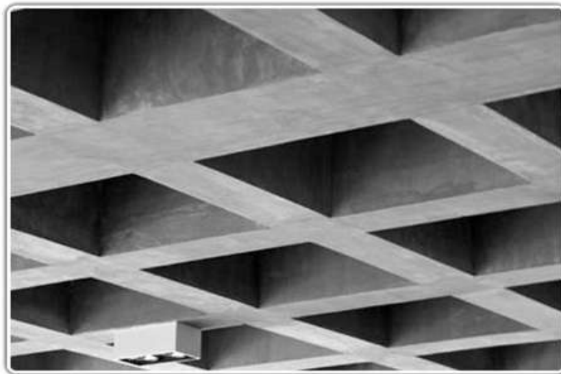
Figure 2: Grid slab
