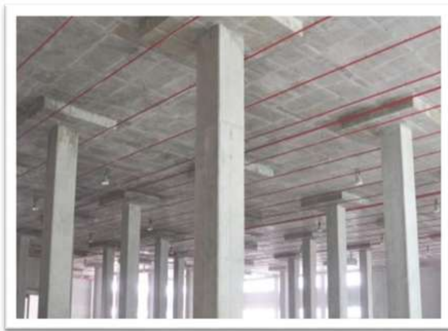
Figure1: Flat slab
