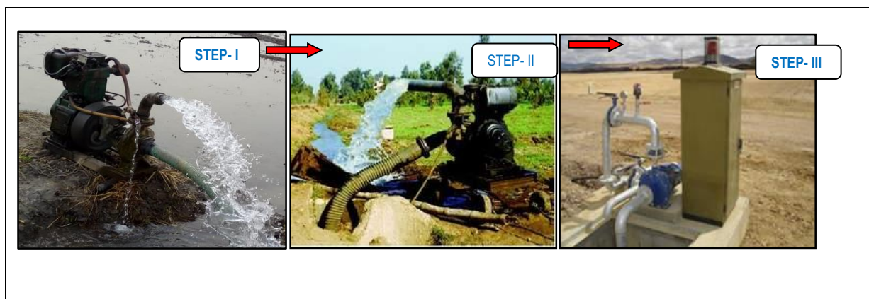
Plate 1C: Modernization steps in an irrigation system.
