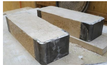
Image (27) shows the completion of casting the mock-up
