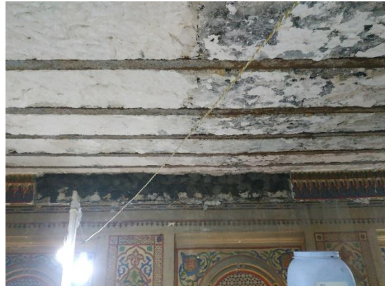
Image (3) show Iron beams from inside the building
