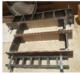
Picture (24) shows preparing molds for casting
