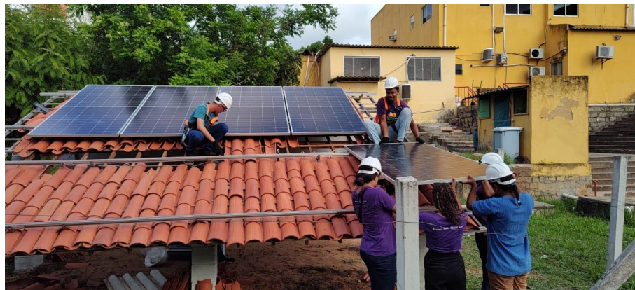
Figure 5 - System assembly photovoltaic on the roof tile didactic ceramics
