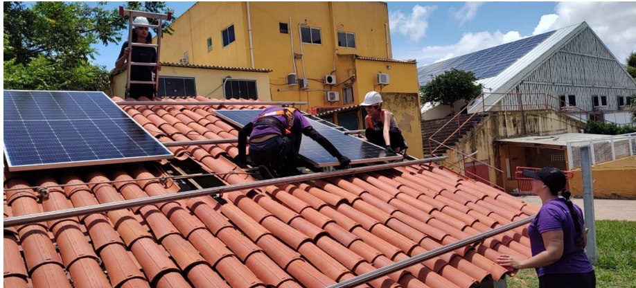
Figure 4 - System assembly photovoltaic on the roof didactic .
