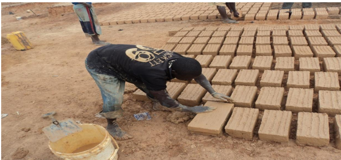
Plate 2. Molded bricks at final stage of production
