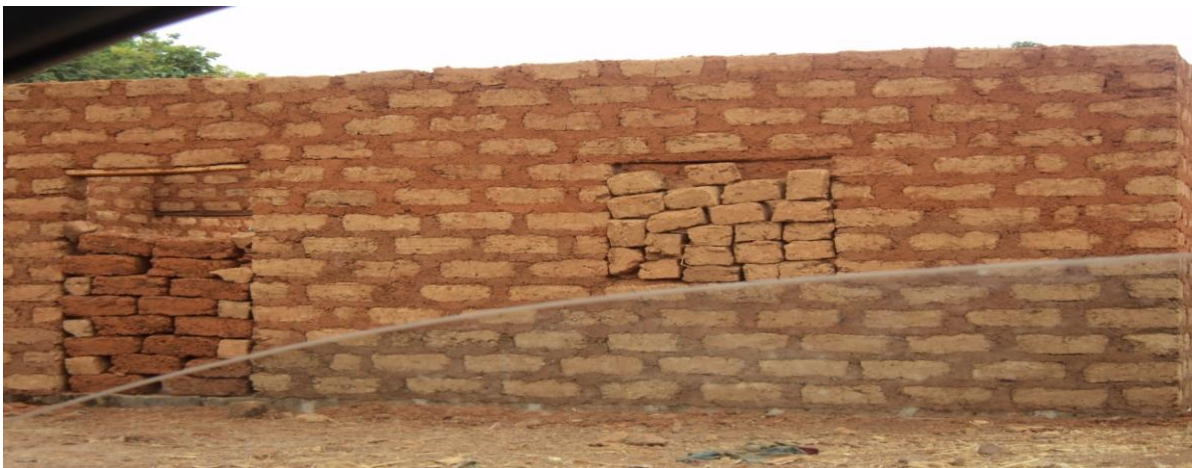
Plate 7. A house under construction
