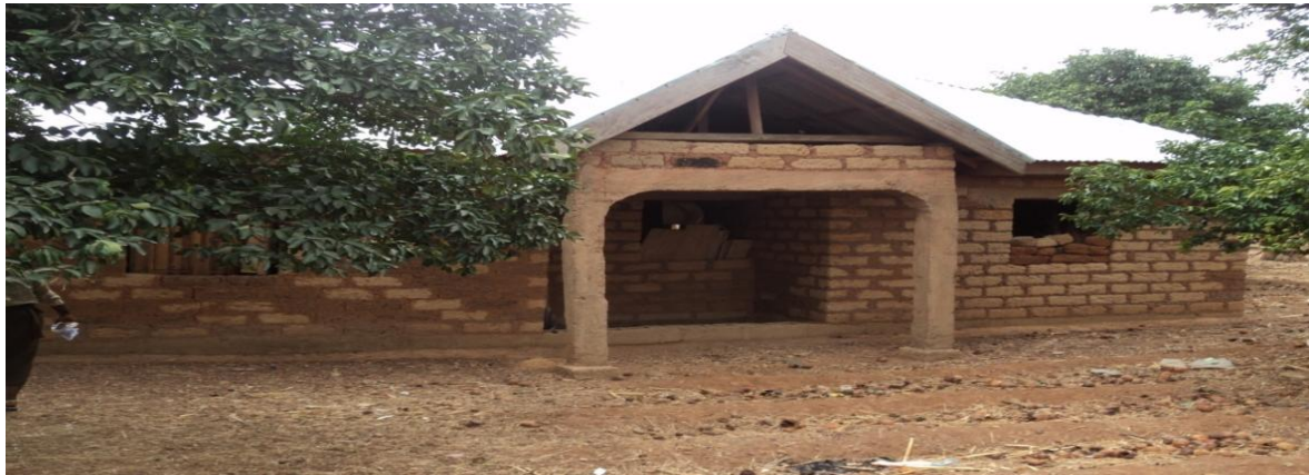
Plate 6. Residential house made with 100% laterite soil
