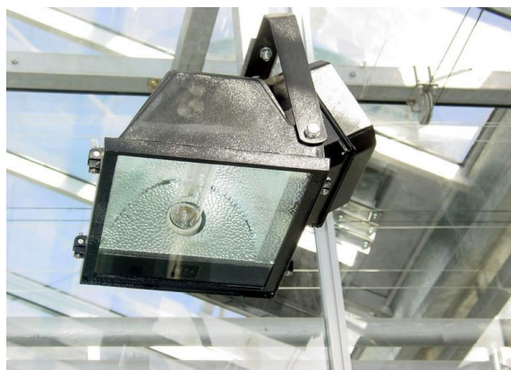
Figure 3 The figure of the sodium lamp to fill light in the greenhouse
