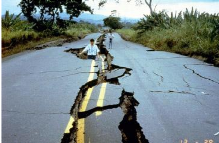
Figure 2. Liquefaction damage after 1991 Costa Rica earthquake [7]
