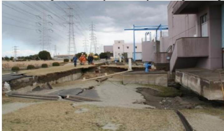
FIGURE 6. LIQUEFACTION DAMAGE AFTER 2011 JAPANESE EARTHQUAKE [11]
