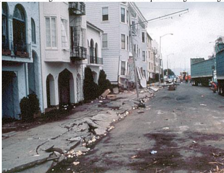
Figure 7. Liquefaction damage after 1989 Loma Prieta [12]
