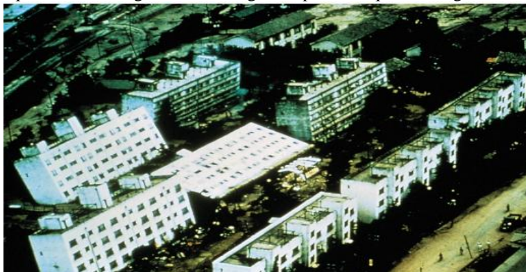
Figure 3. Liquefaction damage after 1964 Niigata, Japan [8]
