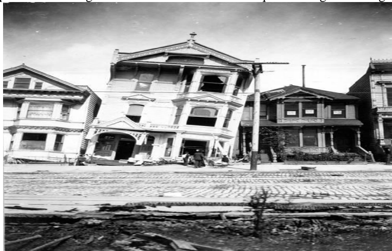
Figure 4. Liquefaction damage after 1906 San Francisco earthquake [9]
