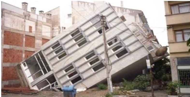
Figure 5. Liquefaction damage after 1999 Turkey earthquake [10]
