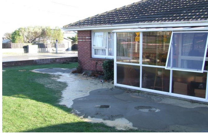
Figure 8. Liquefaction damage after Magnitude 7.0-7.1 Darfield Earthquake (near Christchurch) September 2010 [13]
