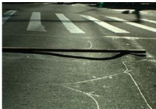
Fig1.1 Rutting phenomenon occurrence in bituminous pavement
