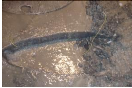
Figure 6. Deformation of the pilot at the depth of 148m.
