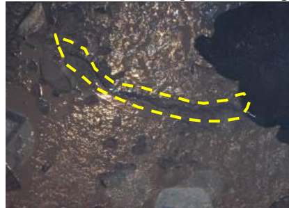
Figure 7. Marking (with broken line) the deformation of the pilot at 154m depth.
