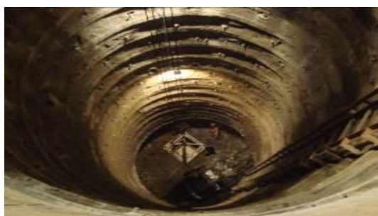
Figure 3. Excavation depth 60m
