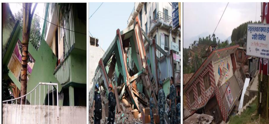
Figure 10. Damages in structural system
