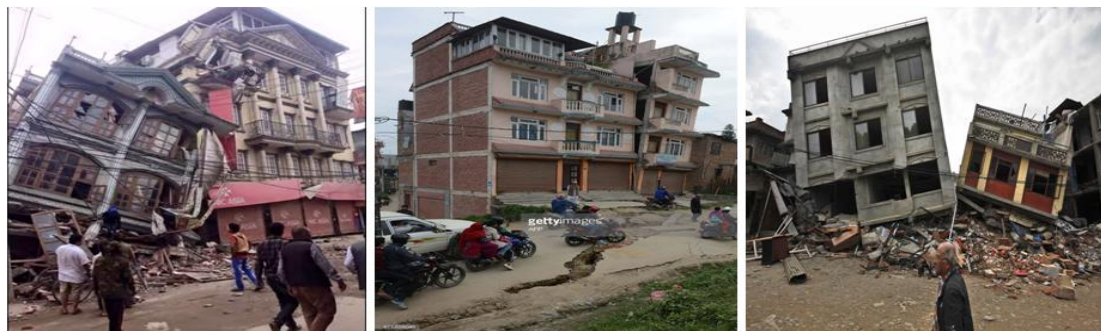
Figure 8. Pounding damages (Source: http://www.haaretz.com/israel-news/1.654075 )
