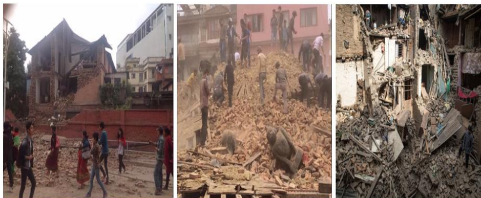
Figure 2. Damages of masonry structures
