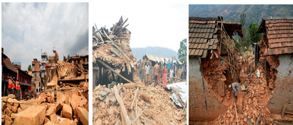
Figure 3. Damages to the poor quality of mortar in stone structures
