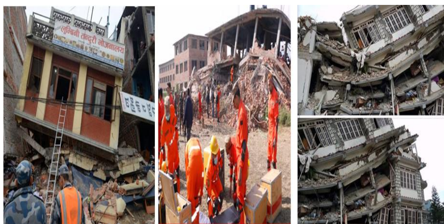
Figure 9. Weak and soft story damages (Source: http://www.haaretz.com/israel-news/1.654075 )
