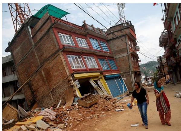
Figure 5. Foundation damage (Source: http://www.ibtimes.co.uk/nepal-buildings-lean-precariouly-aftermath-second-earthquake-photo-report-1501297 )
