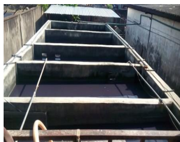
Plate 1: Effluent Treatment Plant (ETP)
