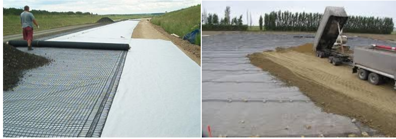
Fig 1.2 Installation of geotextiles
