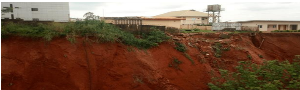
Figure 2.6: The Federal High Court, Awka , Anambra State, Nigeria is under serious gully erosion threat and at the verge of imminent collapse (EnviroNews Nigeria , 2018)
