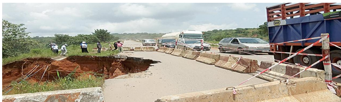
Figure 2. 1: The Ugwuonyeama gully erosion site on Enugu end of the Enugu-Onitsha highway (Njoku, 2018)
