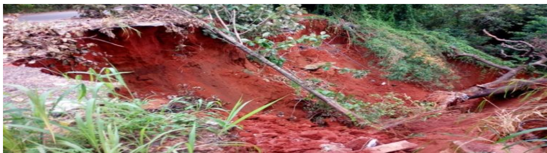
Figure 2.7: Erosion severs Nkpor-Nnobi Road, Onitsha (NAN, 2018)
