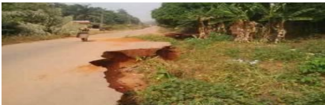
Figure 2.3 Head of gully erosion at a road in Umuaku Uli, Ihiala LGA, Anambra State
