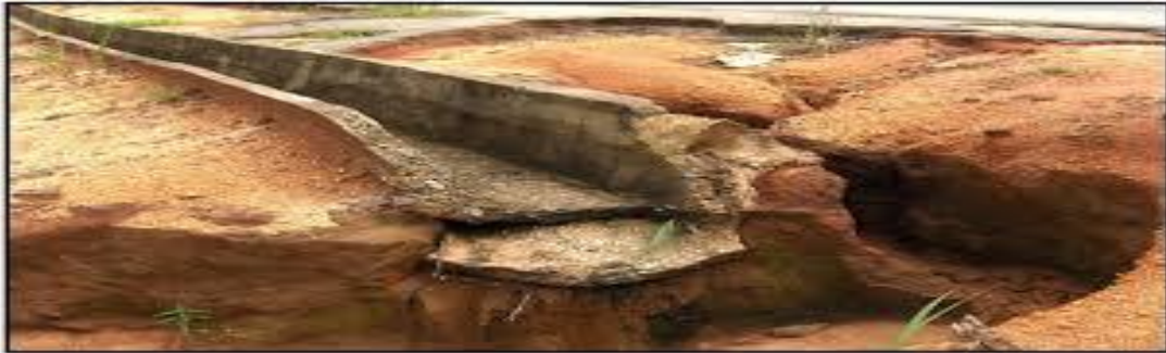
Figure 2.8: Damaged drain channels forming gully erosion at a Nigerian road (Obiadi. et al.2011)
