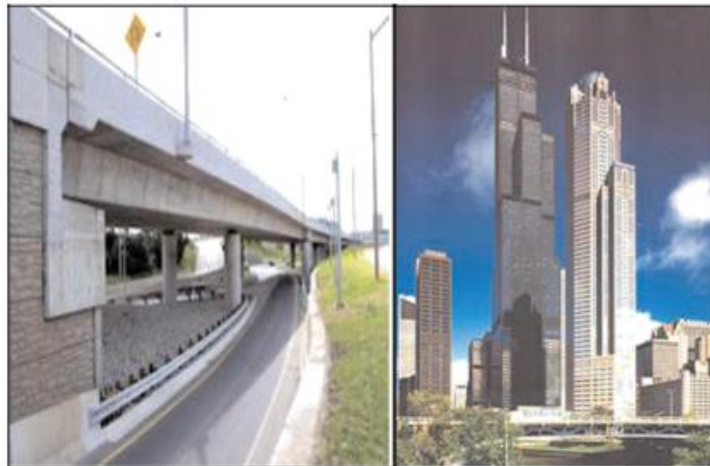
Figure 1: Applications of High Strength Concrete
