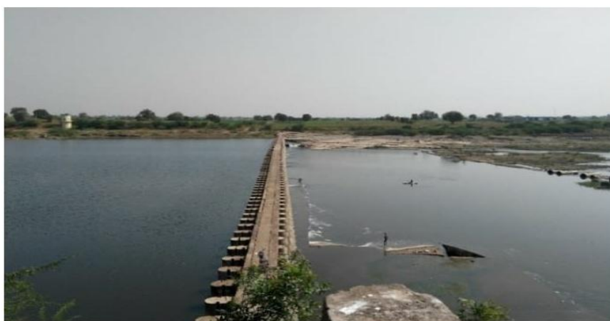
Fig.1.2.c. Saradgi Barrage of Bhima river
