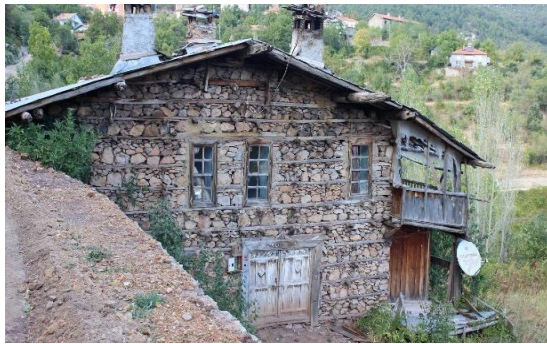
Figure 7: Butonned house sample [13]
