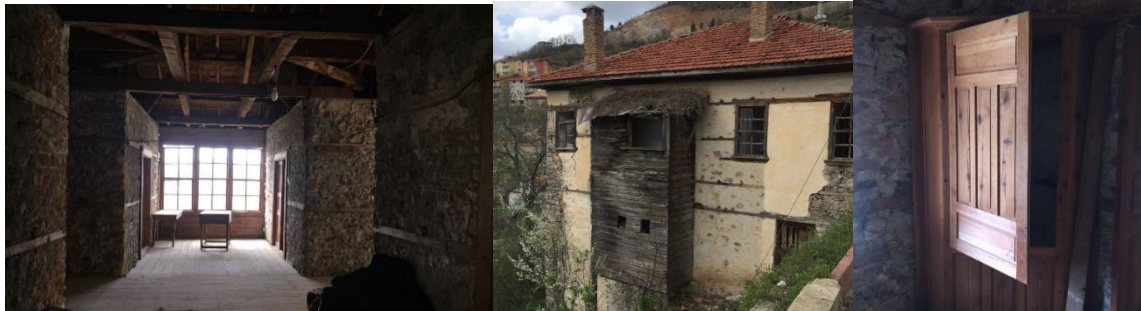
Figure 13: Walls and Floor [13] Figure 14 : Cumba,Windows and Cupboard [13]
