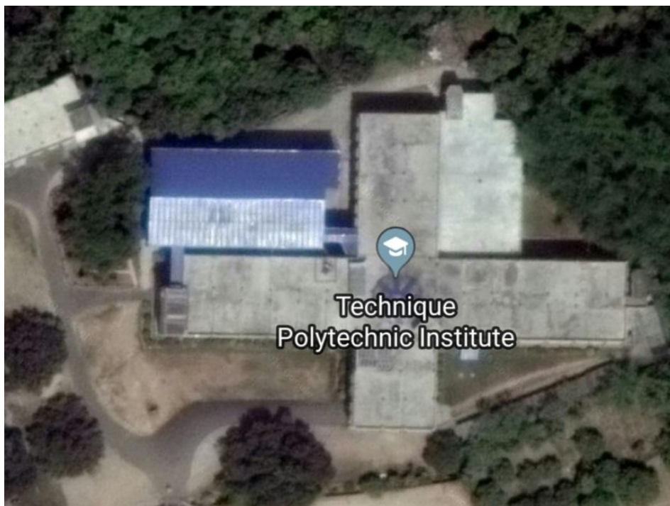
Fig. 1: Roof top view of Technique Polytechnic Institute
