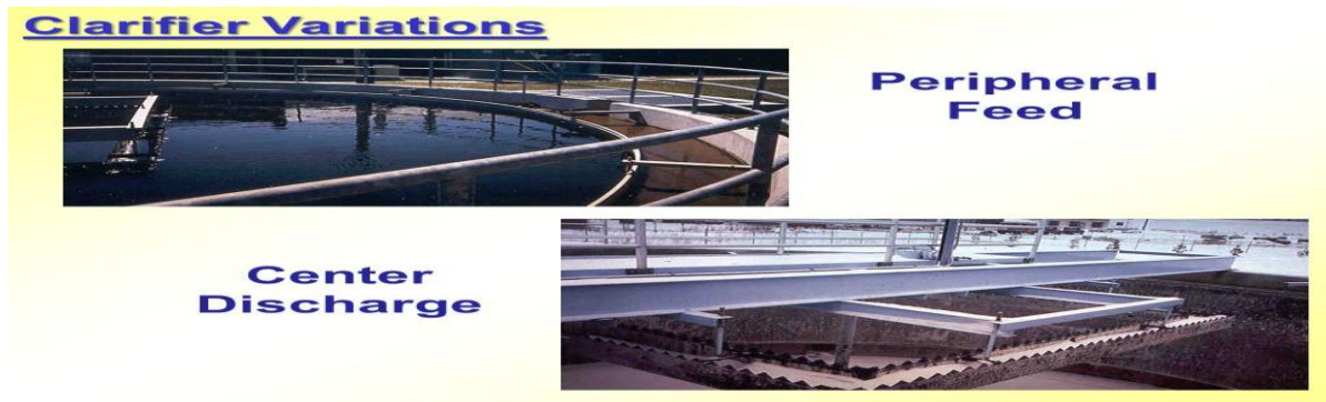
Figure 2 Peripheral feed and center discharge circular clarifier.
