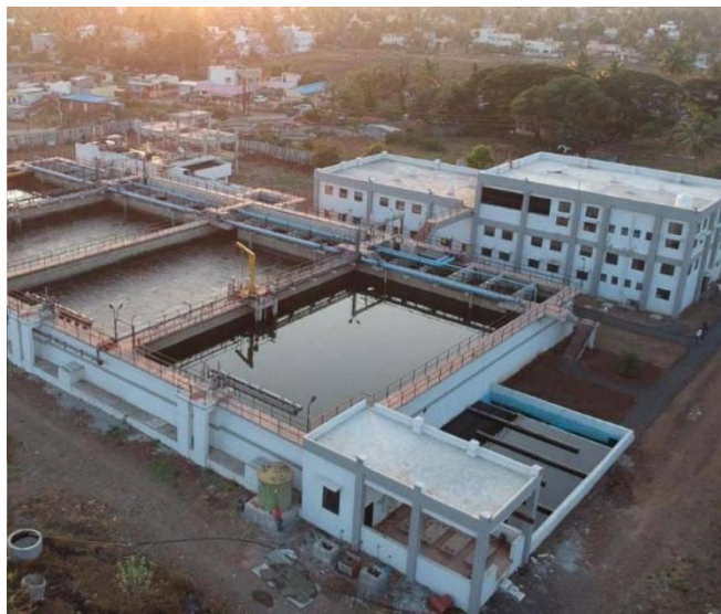
Figure 1.1 Aerial View of Sewage Plant at Sangli Maharashtra
